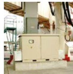
Piller Solid State converter APOJET AJS.
