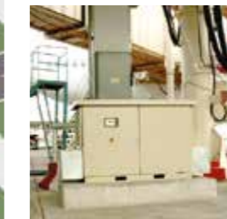
Piller Solid State converter APOJET AJS.
