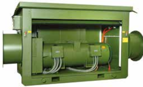
315kVA MG-Set for 400Hz AWACS aircraft supply.
