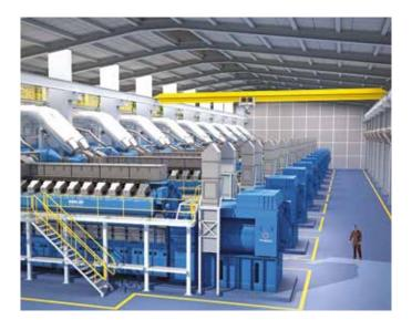
In the case that power is imported or exported a sudden disconnection from the grid in case of a utility outage causes a power imbalance in the microgrid that is compensated by the kinetic energy storage devices of the IPCS until the Bergen engines have balanced their power.
